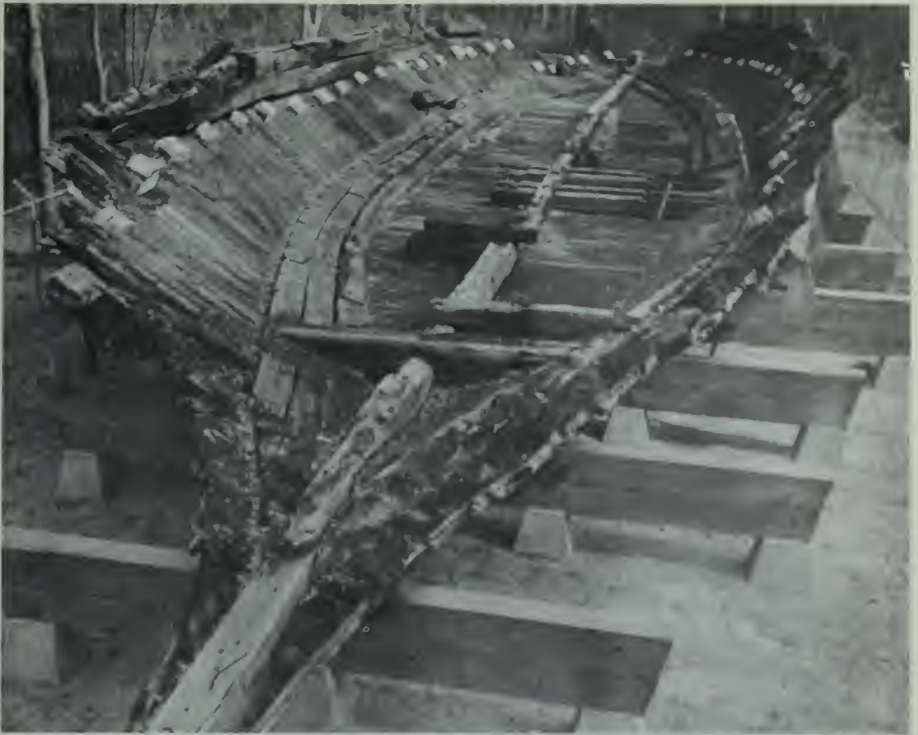
CSS Neuse under reconstruction
